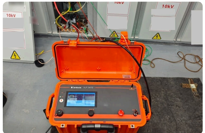
VLF testing on a 10 kV feeder.
