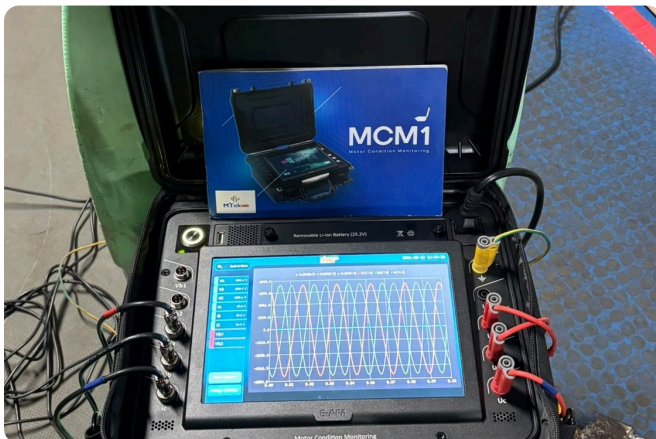
Motor condition monitoring — live three-phase waveforms.
